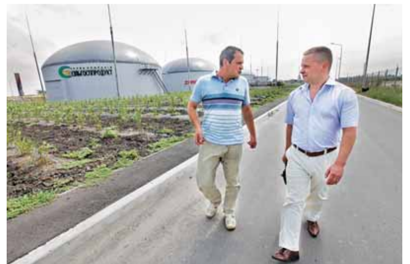
Chief engineer Viktor Ilto (L) of Rokytno biogas plant and its developer Ihor Reddikh, CEO at Zorg Biogas AG, walk on the territory of the station in Rokytno, Kyiv Oblast. (Pavlo Podufalov)
