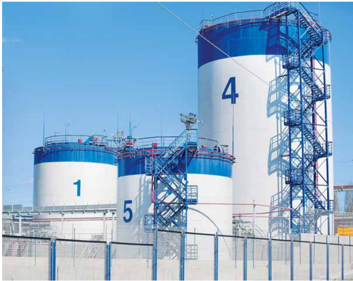
The new terminal for American-based agricultural giant Bunge stands in Mykolaiv on April 12. The company invested $180 million to increase storage capacity to 5 million tons and employs 400 people at the complex for grain and oilseed. (Anastasia Vlasova)
