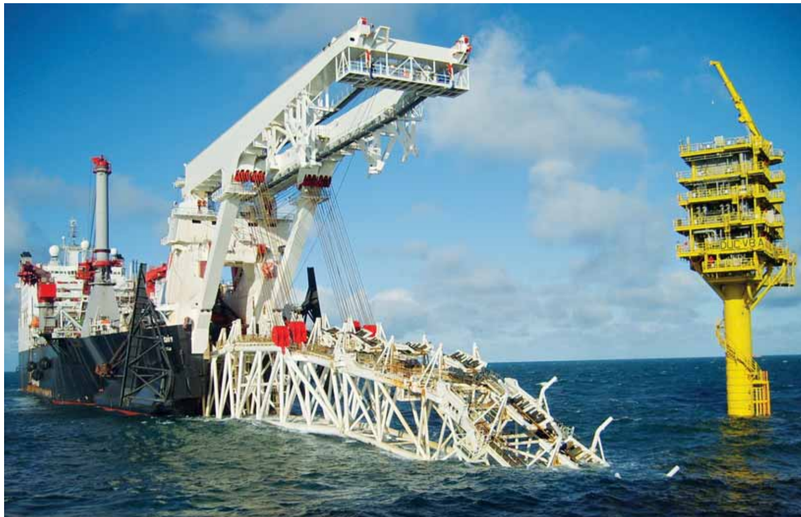
Allseas' Solitaire vessel on Nov. 24 lays pipes for the Nord Stream II pipeline. The $10 billion, 1,200-kilometer project will be capable of transporting 55 billion cubic meters of Russian natural gas across the Baltic Sea to Germany when completed by the end of 2019. (Gazprom)
