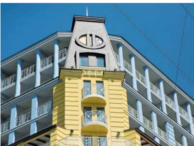
The Podil Prestige apartment complex stands on the corner of Kostantynivska and Nizhny Val in June 2015, after a court put a stay on the building amid an outcry from Podil activists. (UNIAN)
