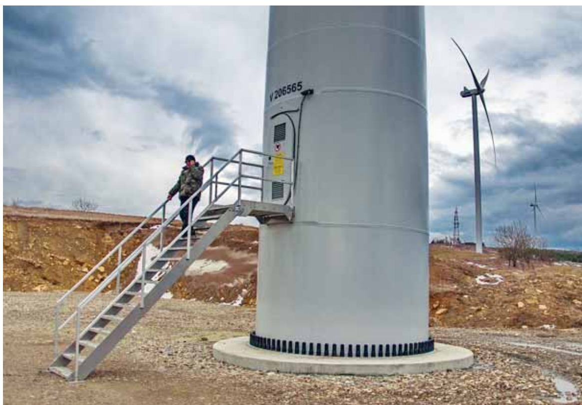
Roman Voloshchak, a power engineer, descends the stairs of one of the four wind turbines at the Eco-Optima wind farm, located near the western Ukrainian town of Staryi Sambir, on Feb. 21. (Yuliana Romanyshyn)
