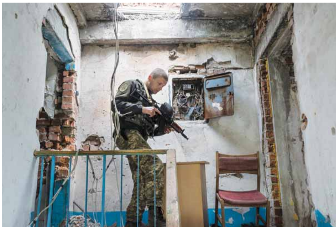
A Ukrainian soldier looks at his helmet while inspecting a heavily damaged apartment building in Donetsk Oblast's Pisky, a town on the frontlines of Russia's war some 700 kilometers southeast of Kyiv, on May 15. (Volodymyr Petrov)
