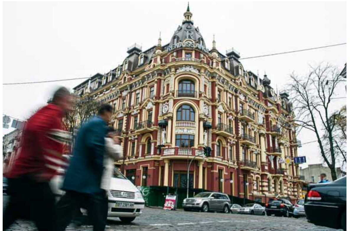
Construction of The Renaissance Hotel near Zoloti Vorota in Kyiv has stalled for years. The building, shown on Oct. 17, 2013 in the picture, is owned by ISTIL Group owner and Kyiv Post publisher Mohammad Zahoor. (Anastasia Vlasova)
