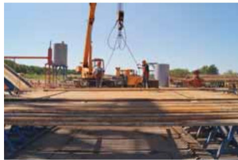
Drilling rig assembly
