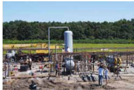
The 2nd degree separator and the divider are already installed
