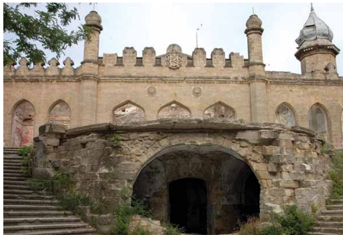
The abandoned building of Kurysy Palace attracts lots of tourists who are looking for some pictorial shots with Moroccan style architectural elements in the background. (Ukrinform)
