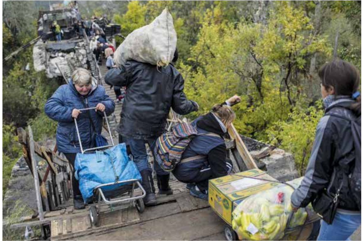
Local civilians cross a heavily damaged bridge at the entry point of Stanytsia Luhanska which leads to the outskirts of the Russian-occupied city of Luhansk on Sept. 26, 2016. (OSCE/Evgeniy Maloletka)
