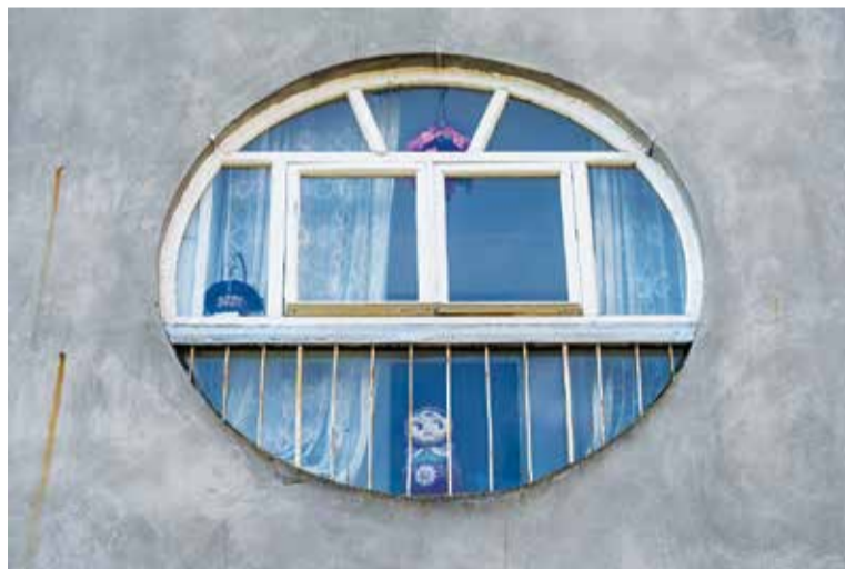
An enclosed balcony in Chernihiv was fitted into a concrete frame. (Balcony Chic / Oleksandr Burlaka)
