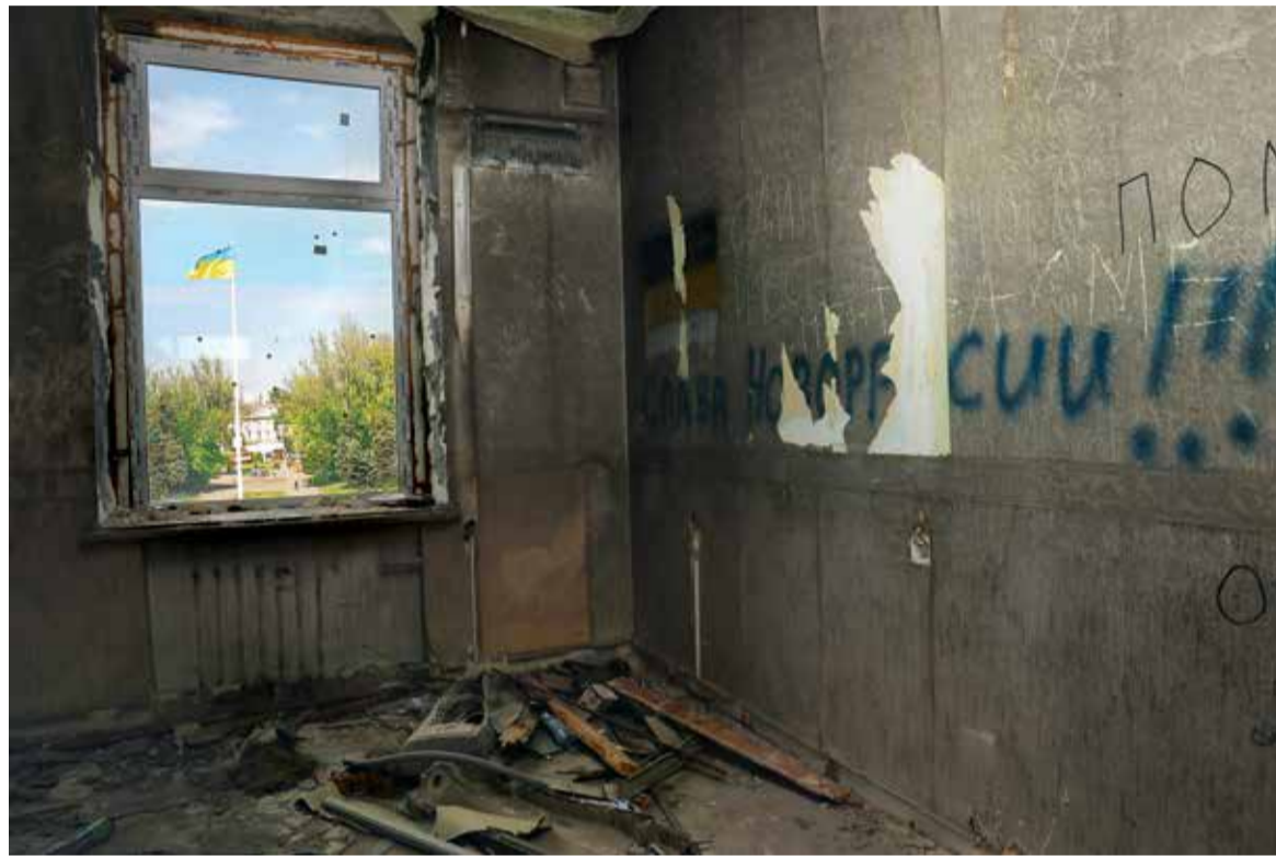
A Ukrainian flag waves outside a window of the Trade Unions House in Odesa, where 42 people were killed in a fire — either directly from the flames or from jumping out windows to escape the blaze — on May 2, 2014. Graffiti on the soot-covered wall reads “Glory to Novorossiya,” a name used in Russian propaganda for southeastern Ukraine. In total, 48 people were killed in Odesa on that day as a result of fights between pro-Ukrainian and pro-Russian activists. (Kostyantyn Chernichkin)
