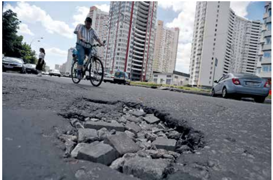
Potholes are a regular characteristic of Ukrainian roads. The country’s roads have been mistreated, underfinanced and neglected for decades, making them some of the worst in the world. But Ukraine’s state road agency, Ukravtodor, is looking for ways to fix the problem. (Oleg Petراسиuk)
