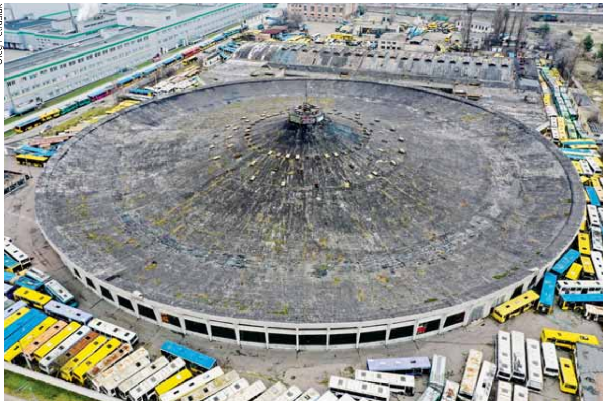
Once considered one of the most innovative structures in the Soviet Union, Bus Depot #7 designed by Vladimir Zinkevich has been defunct since 2015. The sight is one of Kyiv's most extraordinary Soviet architecture creations.
