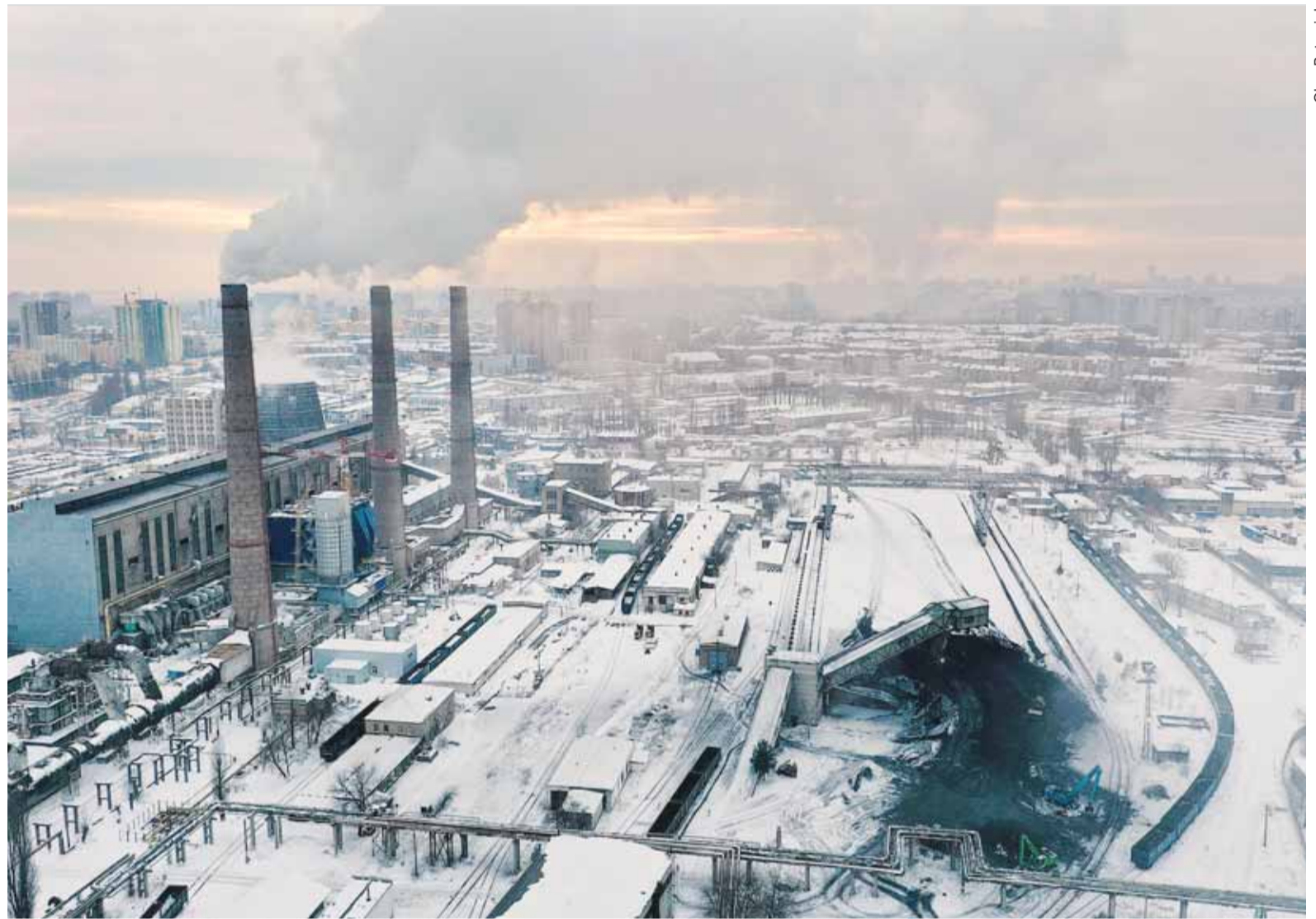
An aerial view of the Darnytska thermal power plant on Feb. 17, 2021. Ukraine's state energy regulator has fined three subsidiaries of Ukraine's largest energy firm DTEK $180,000 for their failure to provide guaranteed coal reserves to thermal power plants in winter, potentially posing a threat to Ukraine's national energy security. DTEK has called the charges against it "baseless" and is going to appeal.
