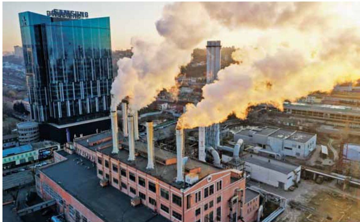
A drone picture shows an aerial view of the DTEK tower and the N°1 Kyivenerho heat supply station in Kyiv on Dec. 7, 2020. DTEK is owned by Rinat Akhmetov, the wealthiest oligarch in Ukraine, and produces the lion's share of Ukraine's coal-fired electricity.
