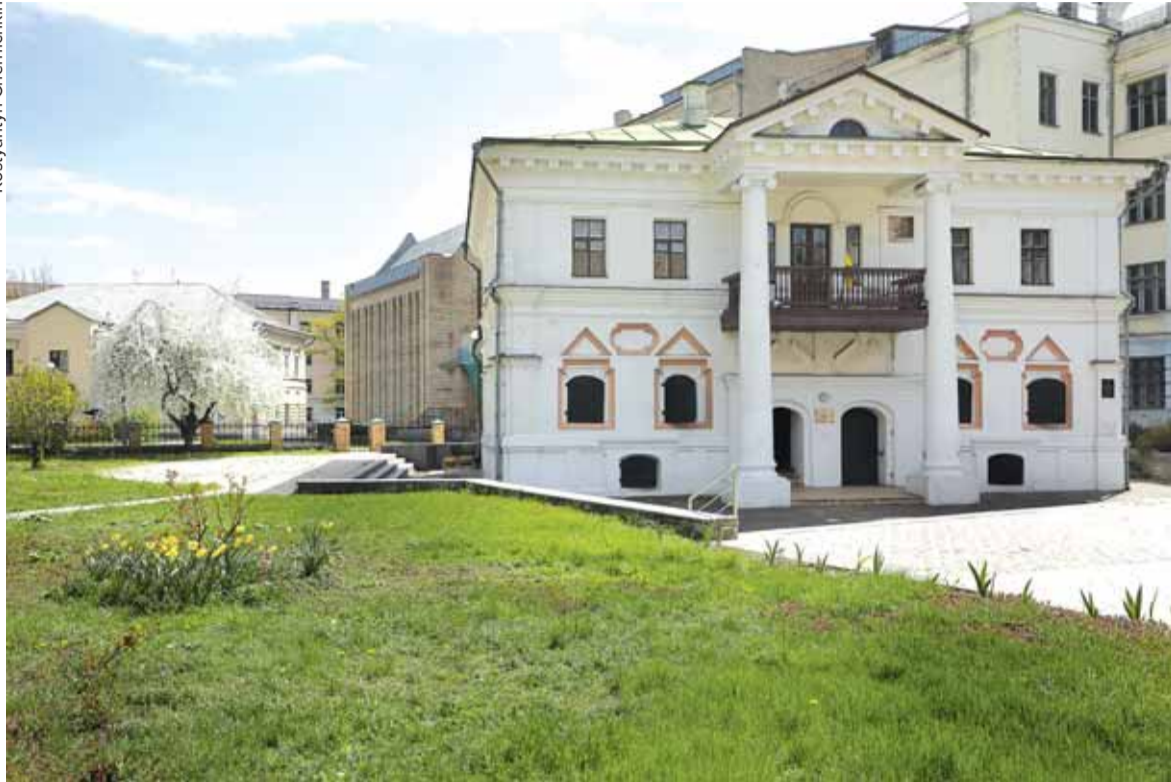
The House of Ivan Mazepa located on 16B Spasskaya St. is one of the few surviving buildings of the Great Podil Fire of 1811, standing in Kyiv for over 300 years. This Ukrainian Baroque styled home is now a museum with more than 9,000 historical items, and exhibits preserving the history and culture of the Cossacks and their Hetmans.
