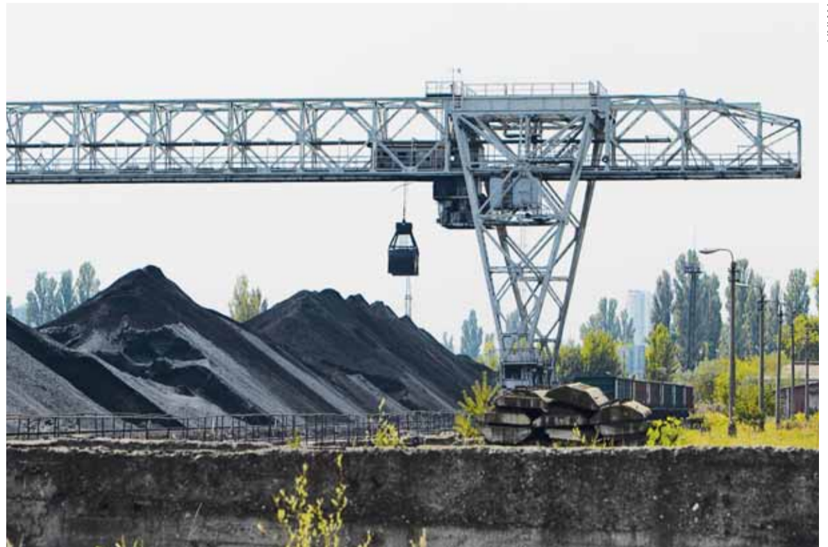
A photo of the Darnytska combined cycle plant in Kyiv, taken on August 12, 2015. The plant is owned by Ukraine's richest oligarch, Rinat Akhmetov, whose power plants are among the biggest polluters in Europe.
