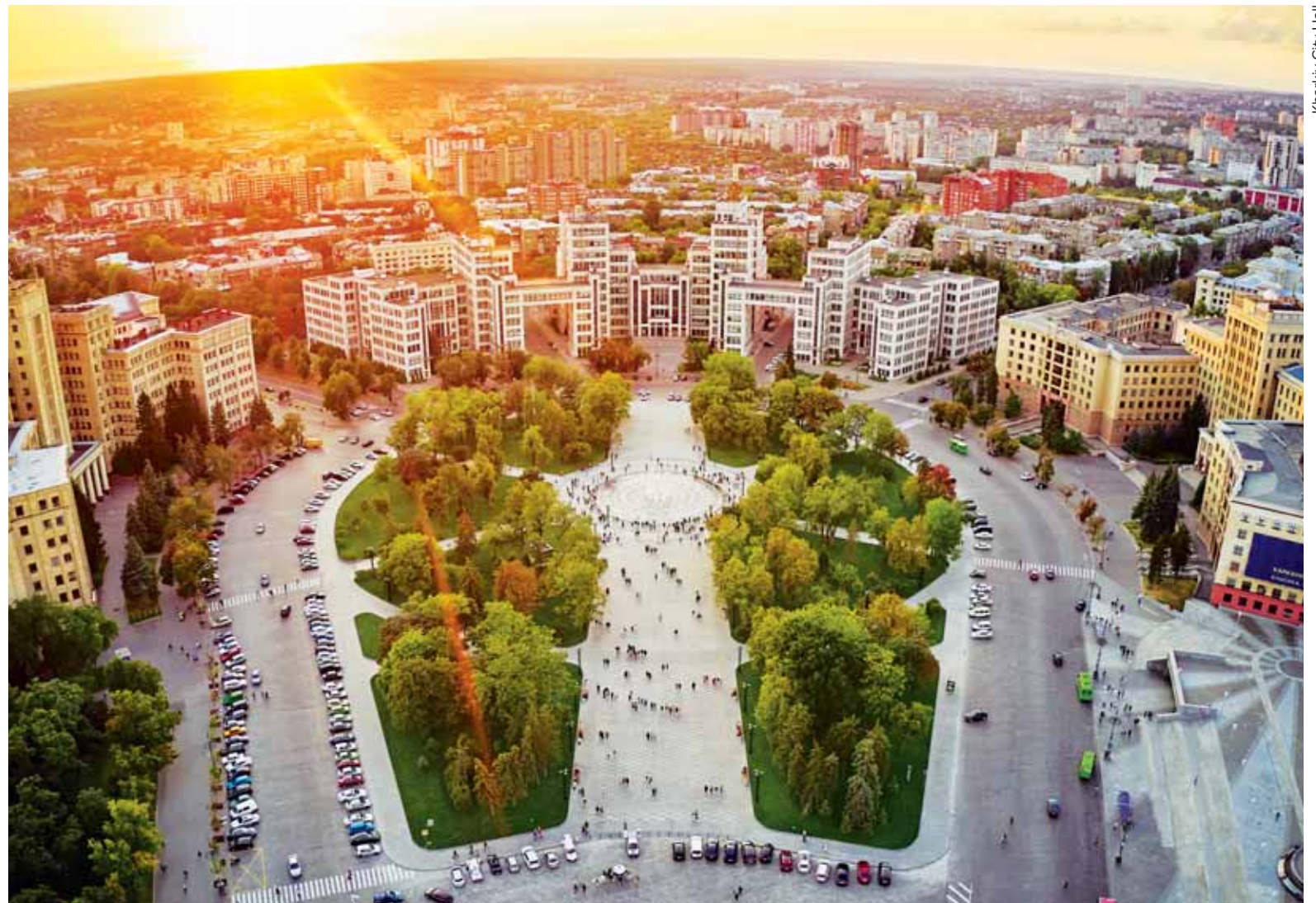
An aerial view of the Svobody (Freedom) Square in Kharkiv shows the constructivist ensemble of buildings of the Derzhprom office center and Vasily Karazin Kharkiv National University. One of Ukraine's oldest educational institutions, Karazin University has a student body of 16,000.
