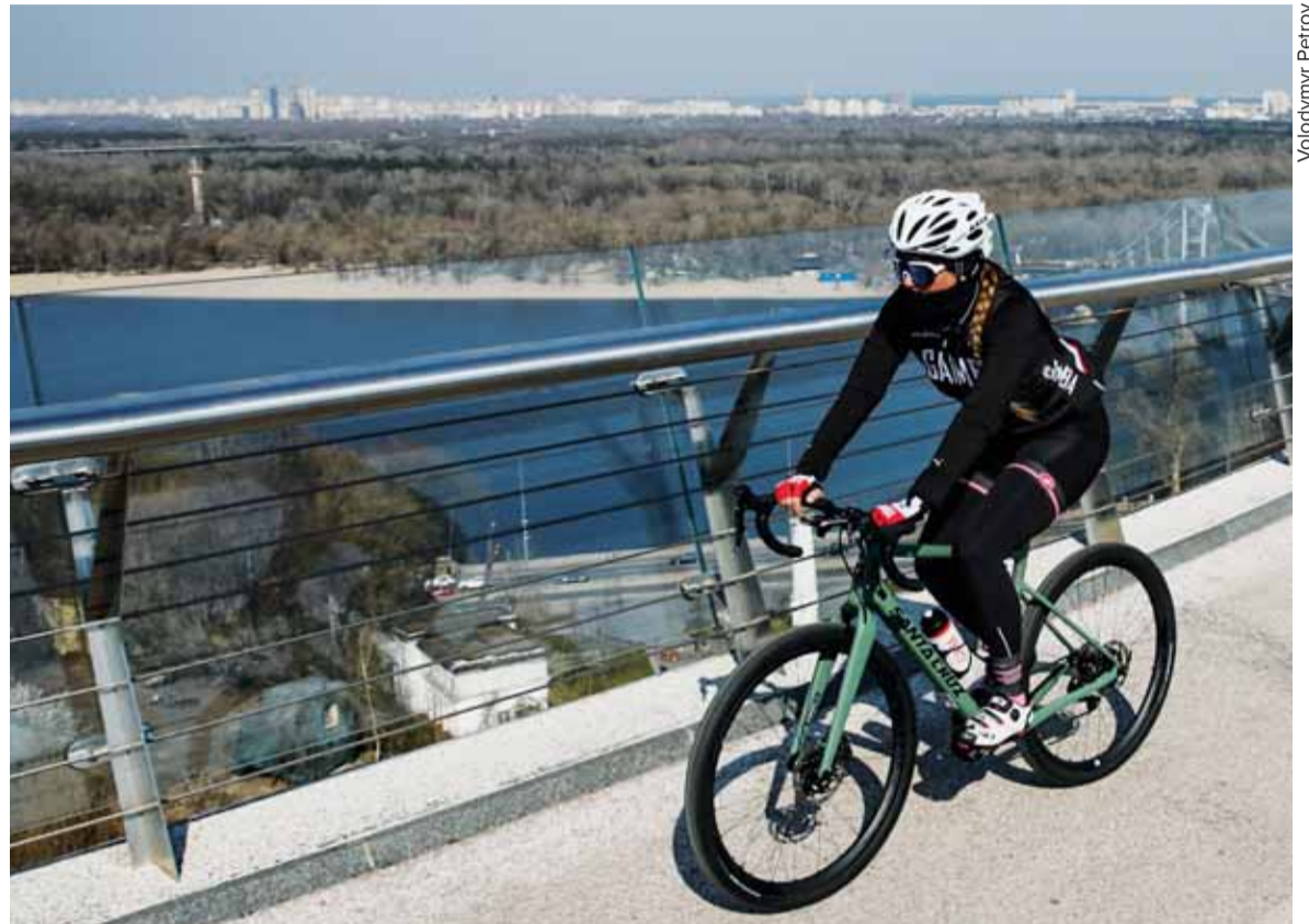
A bicyclist rides along the pedestrian bridge in downtown Kyiv on April 2, 2020. The bridge that connects Mariinsky Park and Volodymyrska Hirka Park is one of the few routes in Kyiv where there is a bike lane.
