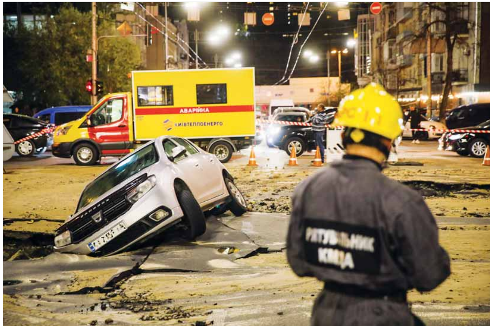
A rescue worker looks over a car stuck in a crater caused by the explosion of a hot water pipe in central Kyiv on Nov. 5, 2019. Sinkholes like these erupt all over the city several times a year due to dilapidated pipes and the lack of funds to properly rehabilitate them.
