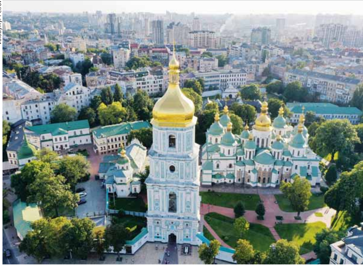
A drone picture shows an aerial view of the Saint Sophia's Cathedral, Kyiv's oldest standing church, a famous historical and architectural monument built in the first half of the 11th century.
