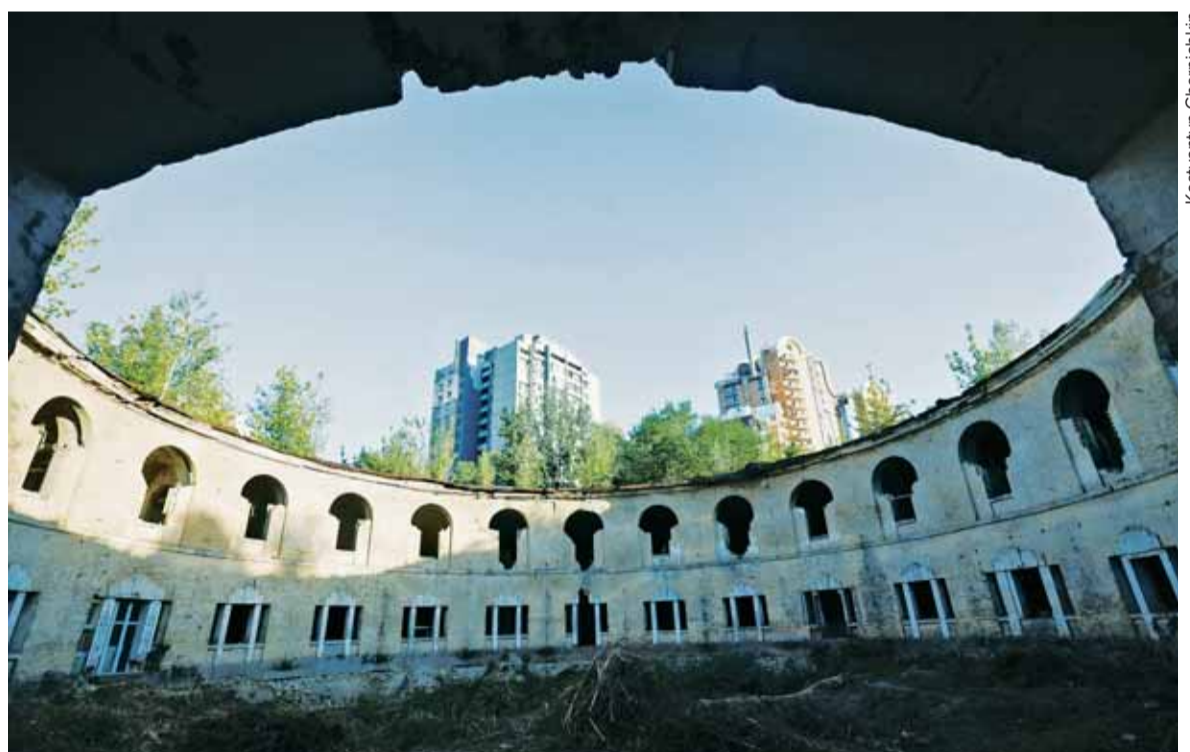
The view from inside the grounds of Navodnitsky tower N°4. Unlike towers 1, 2 and 3, tower 4 has been left to fall into disrepair. In 2017, the Public Cadastral Map of Ukraine suggested that the building would be destroyed. That was later shown to be an error.
