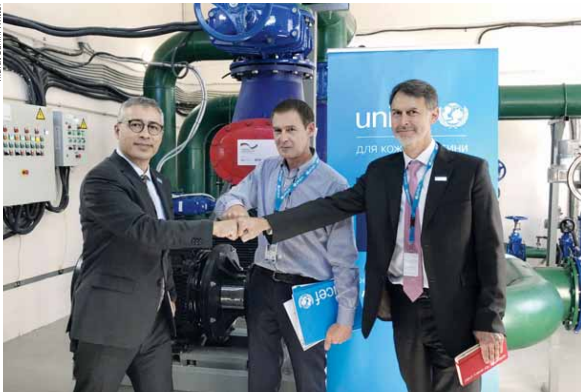
Head of UNICEF Ukraine Murat Sahin (L) fist bumps water and sanitation engineers at a water station in Mariupol, Ukraine on Sept. 17, 2021. Provided by UNICEF with the support of the German government, the new pumping station supplies water for 30,000 people, including four schools and kindergartens, as well as an orphanage.
