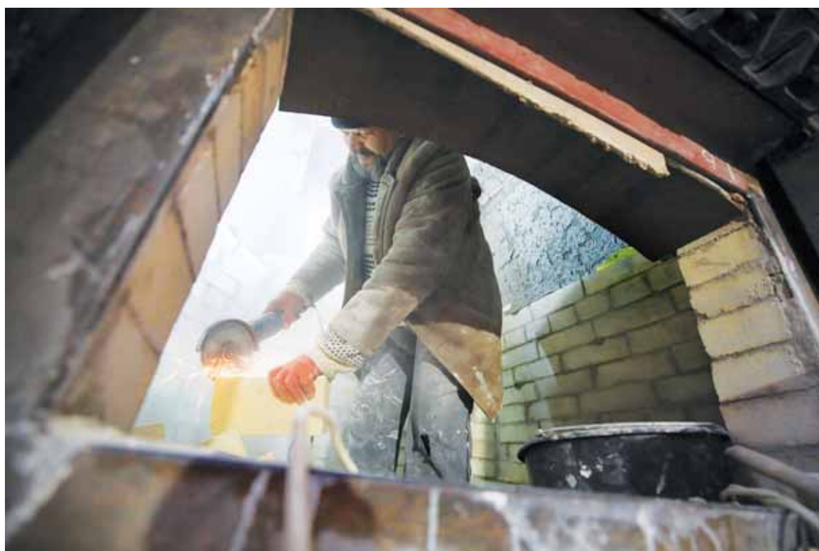
A worker changes heat resistant bricks inside a furnace for the medical waste incineration at the Kyiv's only enterprise that can dispose of hazardous waste, DSL-2010, on Nov. 2 in Kyiv, having used the furnace for several years, the company had to halt it for two months for repair. It plans to put it back into operation by the end of November.
