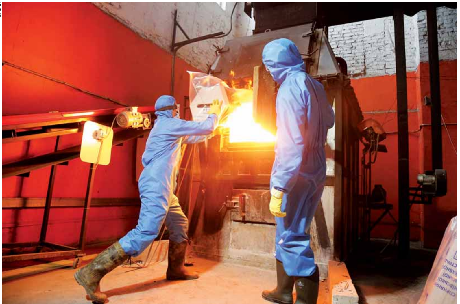
Workers of DSL-2010, the only enterprise in Kyiv that disposes of medical waste, throw used medical masks and gloves into the furnace on May 19, 2020, a few months before the furnace was shut down for repair. Much of the medical waste must be burned in special furnaces at temperatures over 1,200 degrees Celsius to kill bacteria and viruses.
