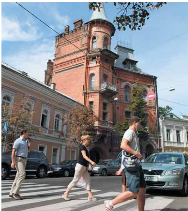
The "House of Gargoyles," one of Kyiv's most beautiful yet neglected and abandoned buildings, is at 1 Yaroslaviv Val. (Ganna Berynk)
