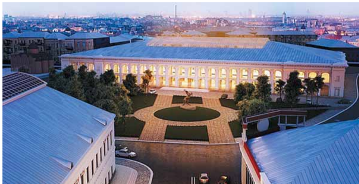
This artist's depiction shows a proposed reconstruction project of Hostynny Dvir. The plan, presented by an architect and Kyiv City Council member Andriy Myrhorodsky, would change the Podil neighborhood building in several ways. Arches will be covered with glass, the third floor rebuilt and the courtyard covered with a glass roof. ( kievcity.gov.ua )
