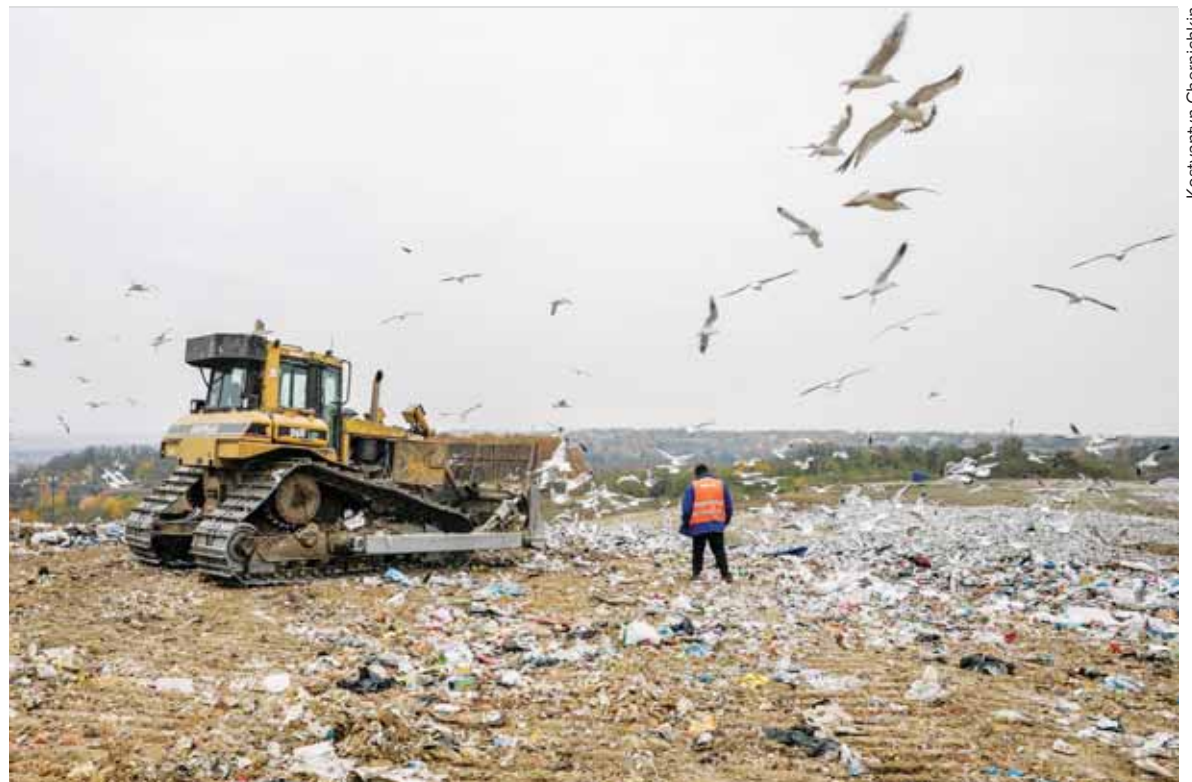
A bulldozer moves garbage around a landfill in Pidhirsia, Kyiv Oblast. Biodegradable plastics such as those made by Bioc could reduce the amount of waste at landfills.
